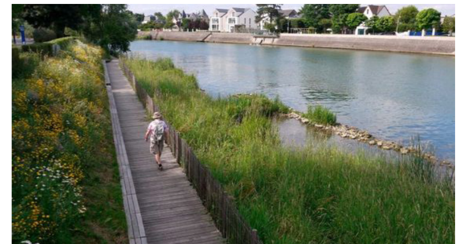
Perreux River Banks by BASE. Photo: BASE
